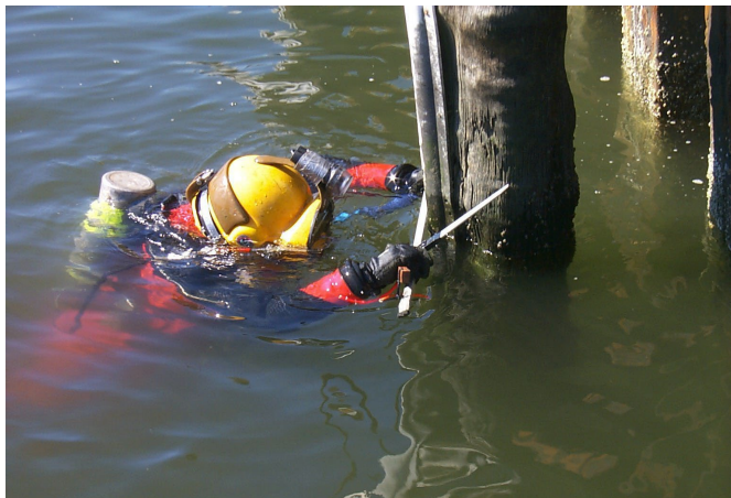
Diver measuring exposed length of timber pile
